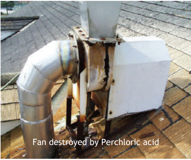
Perchloric acid salts formed on ductwork
