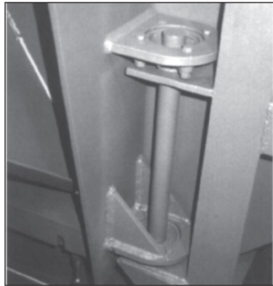
Heavy duty ball bearings provide door support.
