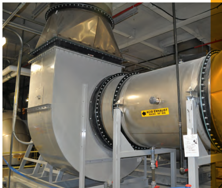
DHK 6000 Fiberglass Exhaust Fan (Global Foundries Semi-Conductor Foundry)
