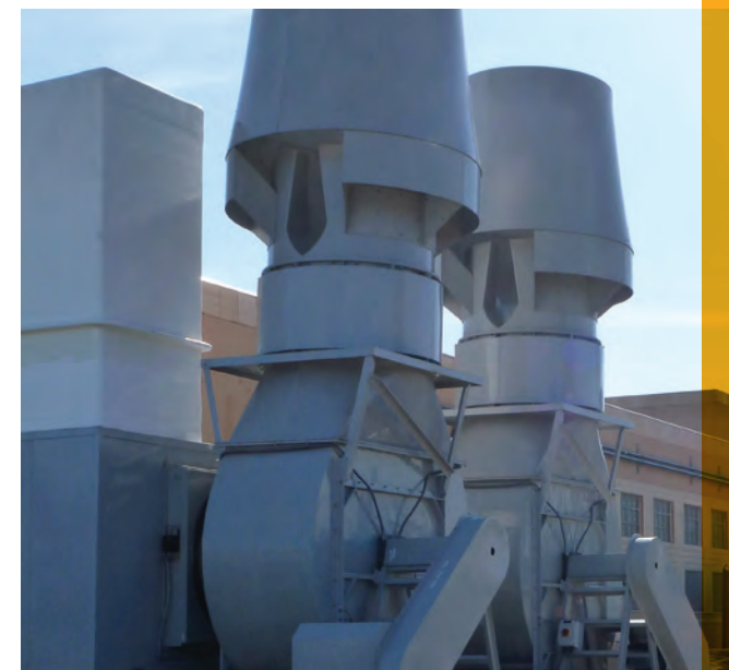
Axijet-F 6000 Fiberglass High Plume Fans (San Francisco Waste Water Treatment Plant)
