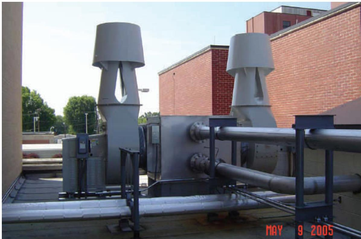
The Axijet fans were designed to run at constant speed regardless of the number of diesels running, or the load. This ensured the design plume height would be maintained. Furthermore, even though the fans would handle hot exhaust, they were selected and powered for air at standard density to accommodate "cold start" testing.
